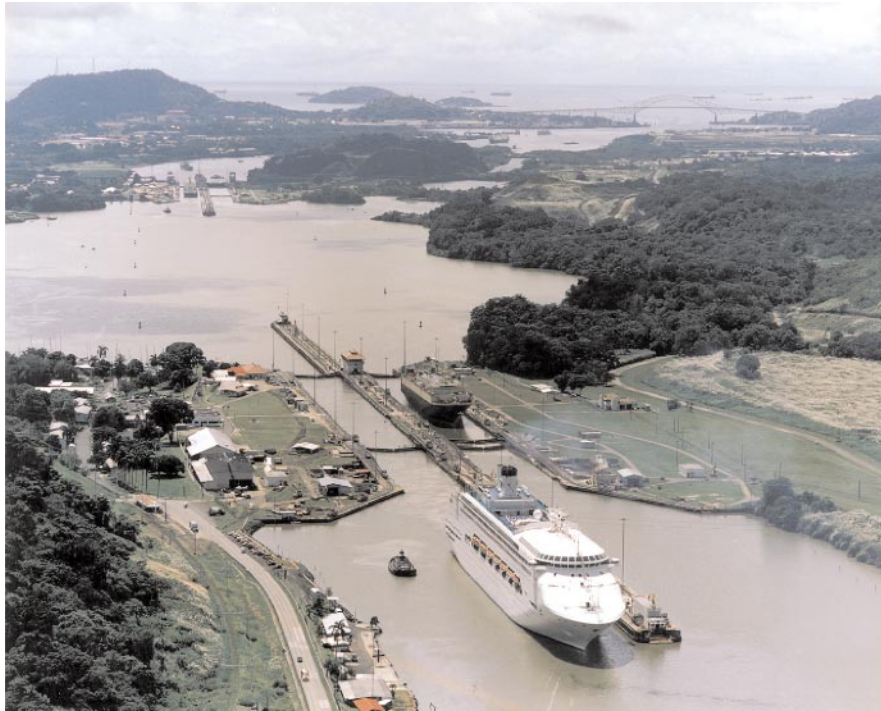
Panama Canal—Pedro Miguel Lock (front), Miraflores Locks (rear), and Thatcher Ferry Bridge from NW
